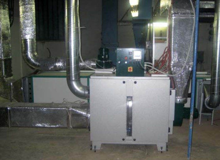
Installed RZ-071 unit with EH-3 control at MILEX cheese factory, Slovak Republic.
